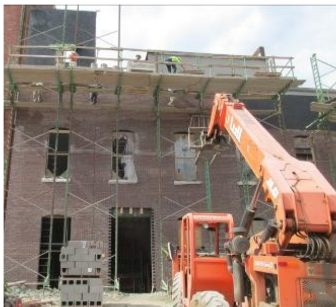
Back of building being bricked.
